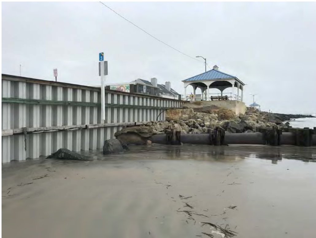
Photo # 2 – View of waterward side of vinyl bulkhead at 3 rd Avenue looking northeast.
