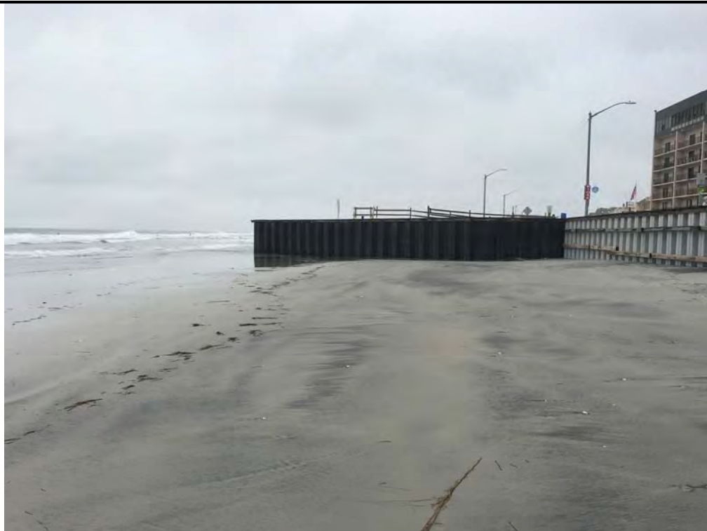
Photo #4 – View of waterward side of vinyl bulkhead and steel bulkhead, and former dune area at 4 th Avenue looking southwest.
