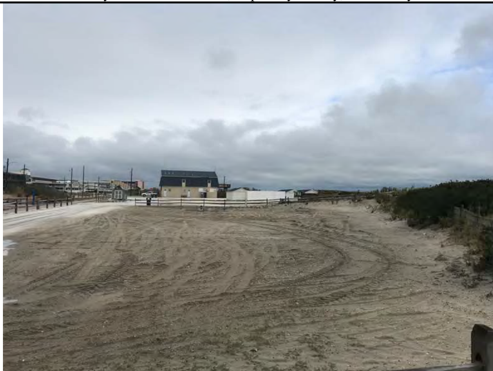
Photo #19 – View of proposed bulkhead location at 16 th Avenue looking northeast at the Beach Patrol Building.
