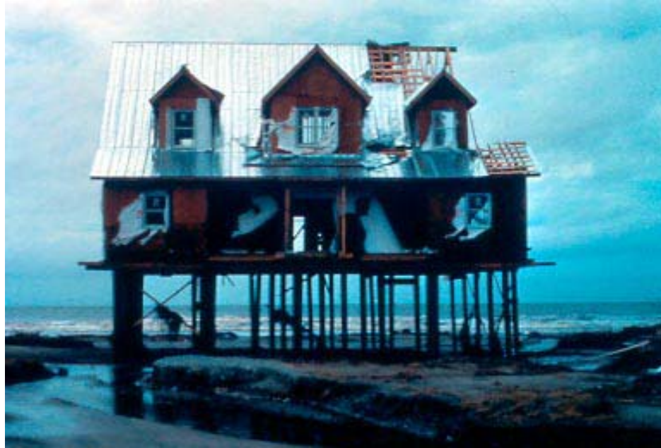
Figure 7. Extensively damaged home south of Litchfield Camp, South Carolina as a result of Hurricane Hugo. In addition to the heavy damage to the structure of the building itself from wind and wave damage, note evidence of wave-induced erosion and scour under the house and around pilings and creation of channels toward the viewer (Photo courtesy of Dr. MaryJo Hall).
