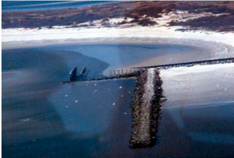
Figure 54. Aerial photograph showing advanced terminal groin effects, Stone Harbor Point, NJ in early March 1984 (before the late March storm). Erosion caused by terminal rock groin in foreground has caused erosion in an arcing pattern behind the structure actually flanking it. Subsequently, the entire Point eroded away (dune field and spit visible in background). (Photograph by Dr. Susan D. Halsey)
