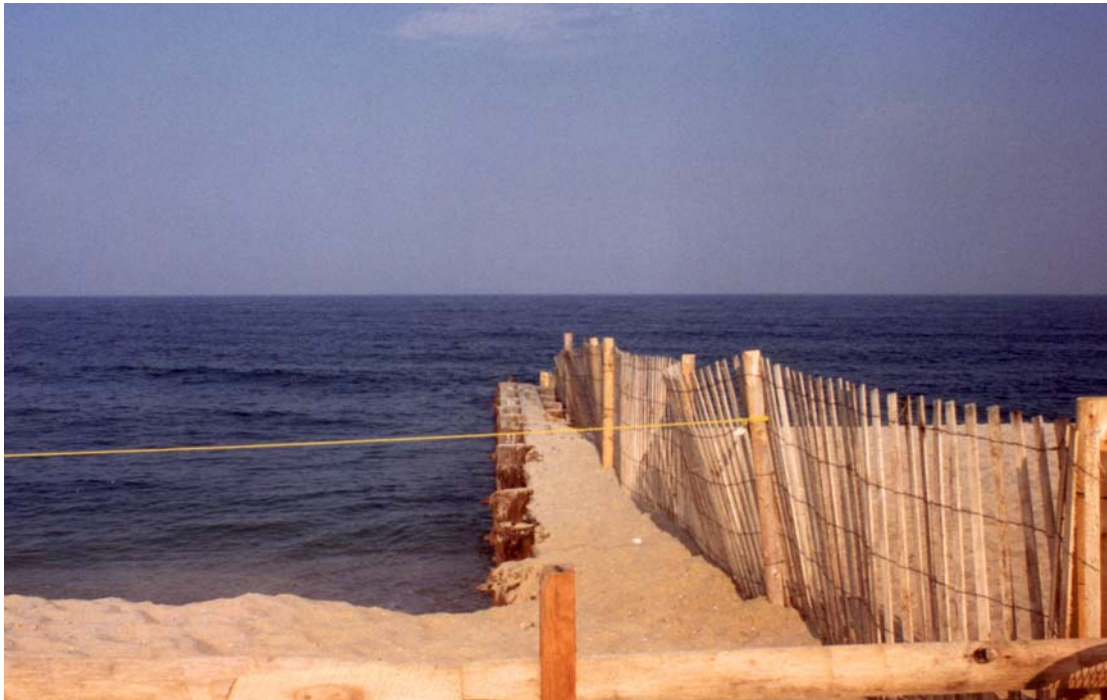
Figure 24. Localized erosion on the downdrift side of a timber groin in Manasquan, NJ, caused by prolonged unidirectional sediment transport (Photograph by Dr. Michael S. Bruno).
