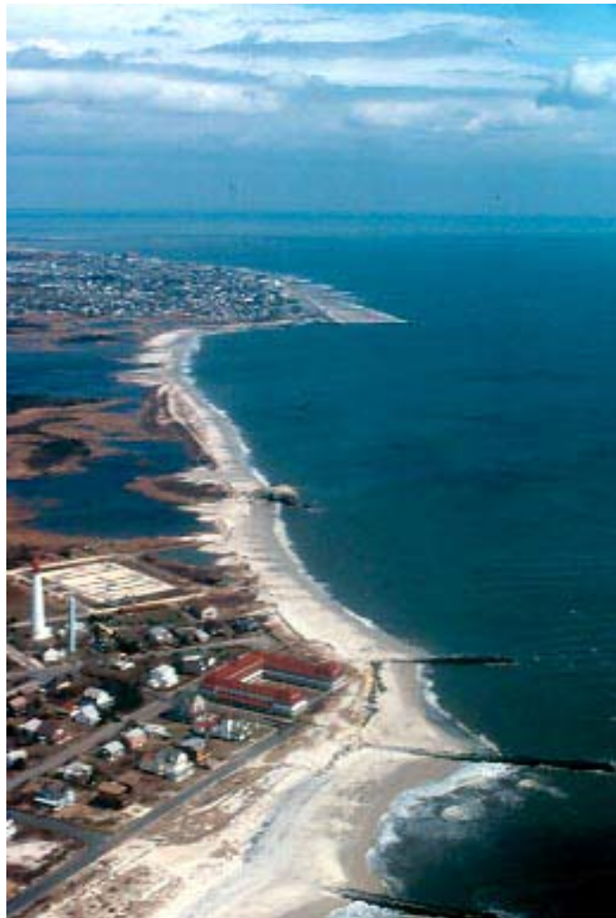
Figure 55. Aerial photograph of the “Cape May Meadows” area, Cape May Point, NJ after the March 1984 storm. Terminal groin effect from Cape May City (in top distance) has eroded the meadows area in the classical arced pattern. Note extensive washover fans with sand reaching into the ponds and salt marsh, and old World War II bunker in surf zone. Originally the bunker was approximately 1000 feet behind the dune line when built. (Photograph by Dr. Susan D. Halsey)
