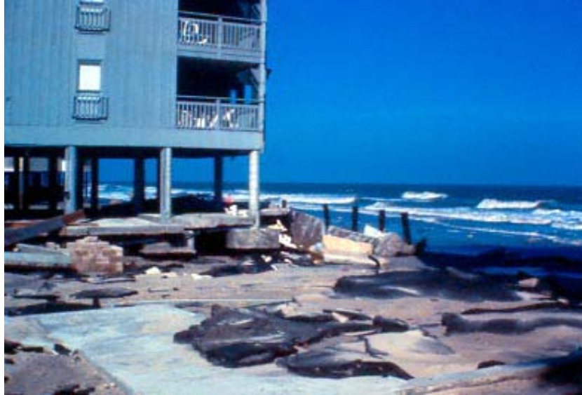
Figure 22. Hurricane Hugo induced failure of an ocean front bulkhead in Myrtle Beach, South Carolina that resulted in substantial damage to a condominium building (Photo courtesy of Dr. MaryJo Hall).
