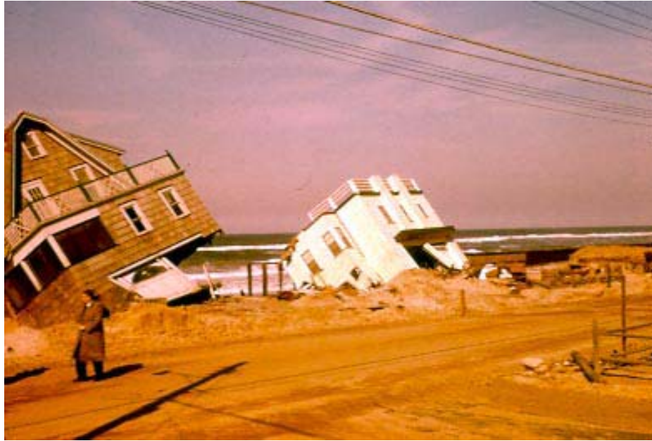
Figure 8. Brant Beach section of Long Beach Island, New Jersey after the March, 1962 storm. Houses with regular foundations undermined by wave scour on the oceanfront, cinder blocks failed and houses tipped down the scarp (cliff) toward the ocean. The number of damaged homes from this storm led to FEMA subsequently requiring houses in specific zones to be built on pilings (Photo by Al Chance, courtesy of Dr. Susan D. Halsey).
