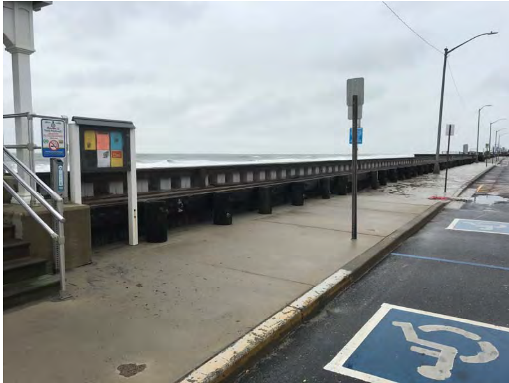
Photo #1 – View of landward side of vinyl bulkhead at 3 rd Avenue looking southwest.
