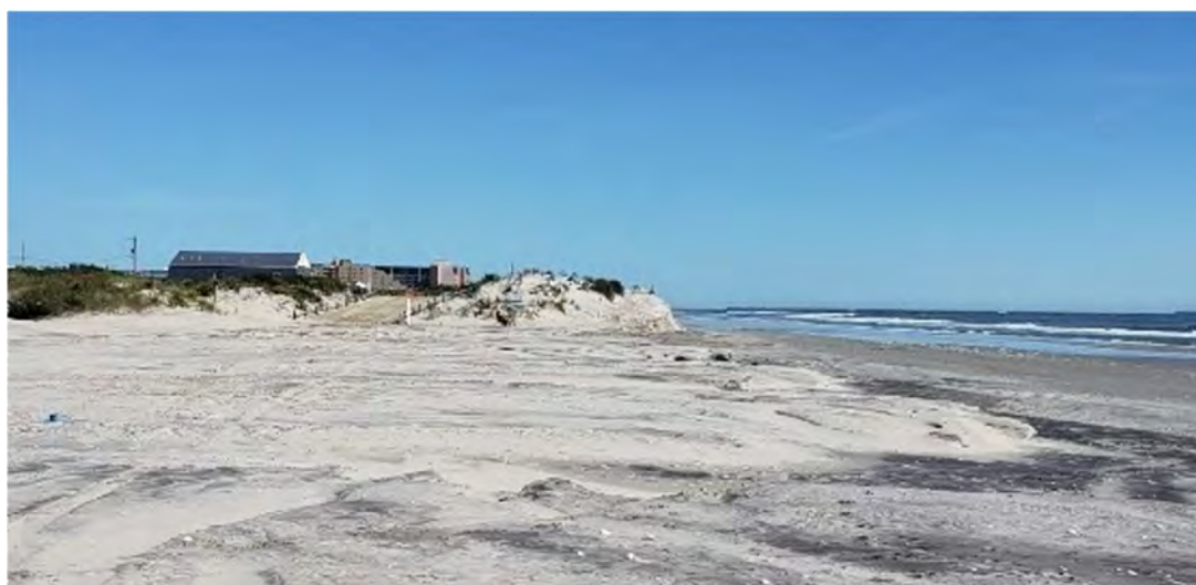
Figure 4: Ground level view looking north at the North Wildwood Beach Patrol Headquarters after the passage of Hurricane Ian.
