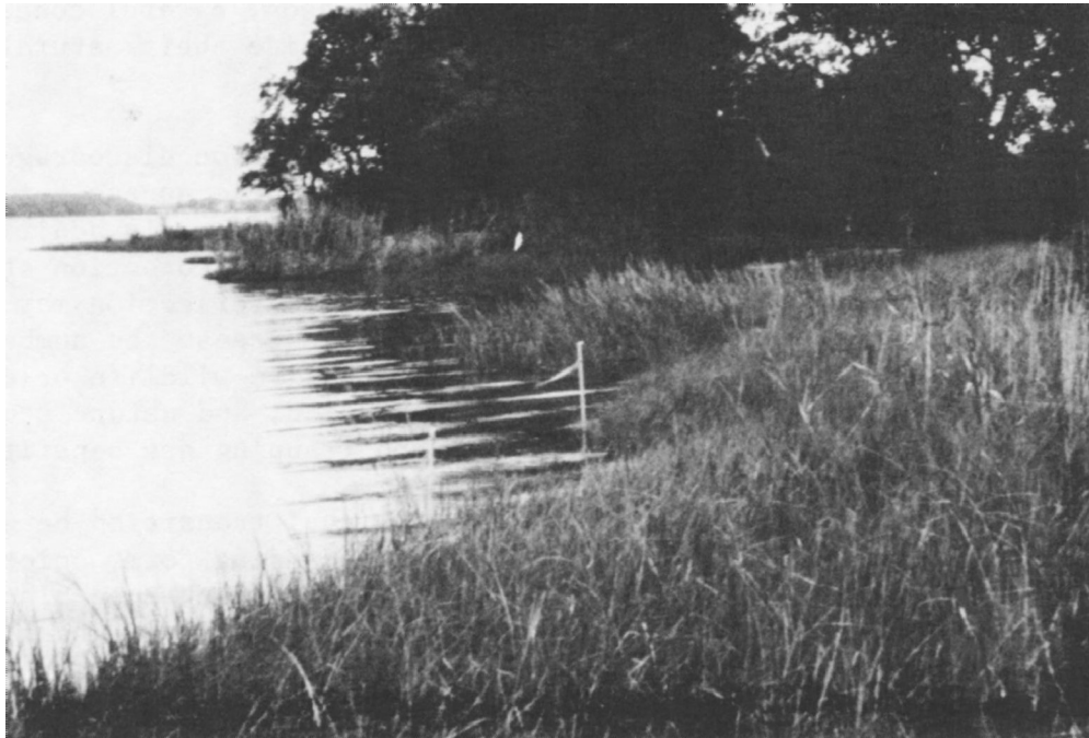
a. Vegetative erosion control project (Maryland)
