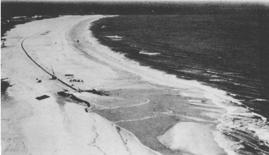
Figure 4-2. Beach nourishment operation, Mayport, Florida (courtesy of US Army Engineer District, Jacksonville)
