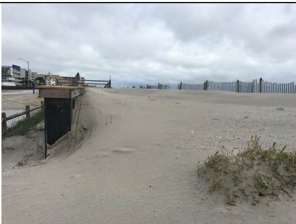
Photo #16 – View of steel bulkhead and location of former wetland at 13 th Avenue looking northeast.
