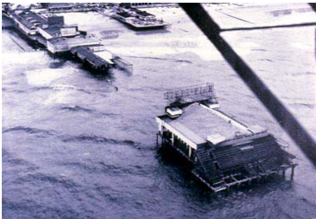
Figure 11. Damage to Atlantic City's Steel Pier from the March, 1962 storm. Note missing center portion removed by wave uplift during the height of the storm (Photo courtesy of Dr. Susan D. Halsey).
