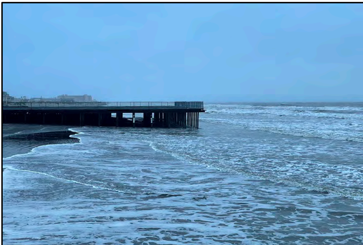
PHOTOGRAPH 3. View north of the 24 th Avenue pier terminus and absence of beach berm waterward of the pier end, which precludes the sand backpassing truck route.
