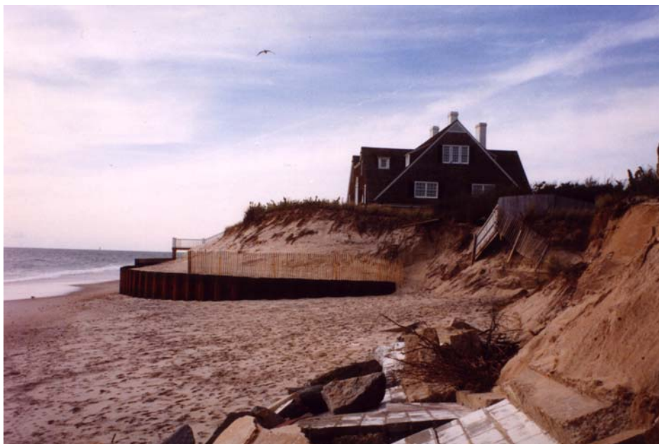
Figure 56. A sheet metal bulkhead installed to prevent the undermining of a dune and adjacent home. Bulkheads exposed to direct wave attack can result in the loss of sediments fronting the structure (Photograph by Dr. Michael S. Bruno).
