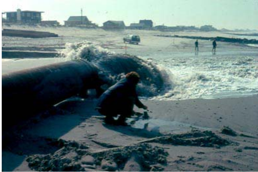
Figure 37. Emergency beach nourishment project underway on Long Beach Island, NJ, March 1979. Sand from Barnegat Inlet was pumped through pipes at two locations; one further up the beach profile and one near the proposed low tide line. Note pipes on upper beach waiting for placement near the dune scarp created by a trio of northeasters in the winter of 1978-1979. After the nourishment project, groins seen in this photograph were not visible. (Photograph by Dr. Susan D. Halsey)
