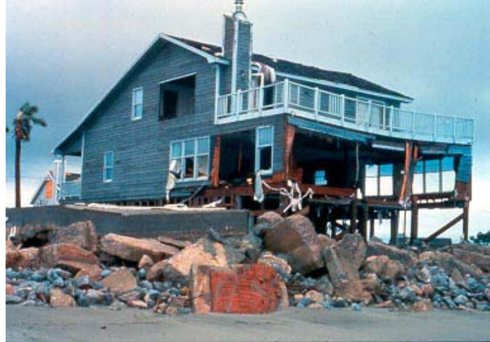
Figure 16. Extensive wind damage to house near Myrtle Beach, South Carolina as a result of Hurricane Hugo. Note loss of not only front plate glass windows, but also loss of side windows (Photo courtesy of Dr. MaryJo Hall).
