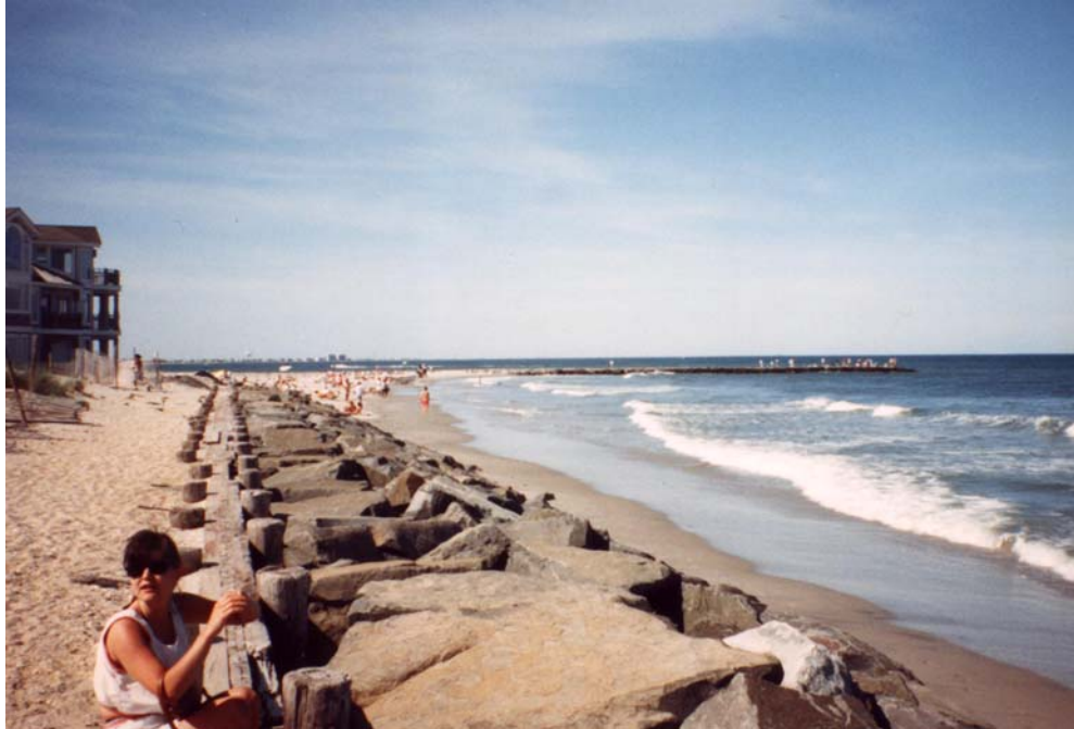
Figure 59. Rock revetment fronting a timber bulkhead along the Avalon, New Jersey coastline (Photograph by Dr. Thomas O. Herrington).
