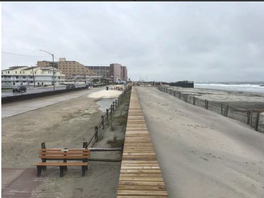
Photo #13 – View of timber cap and steel bulkhead at 9 th Avenue looking northeast showing location of former wetlands/dune.
