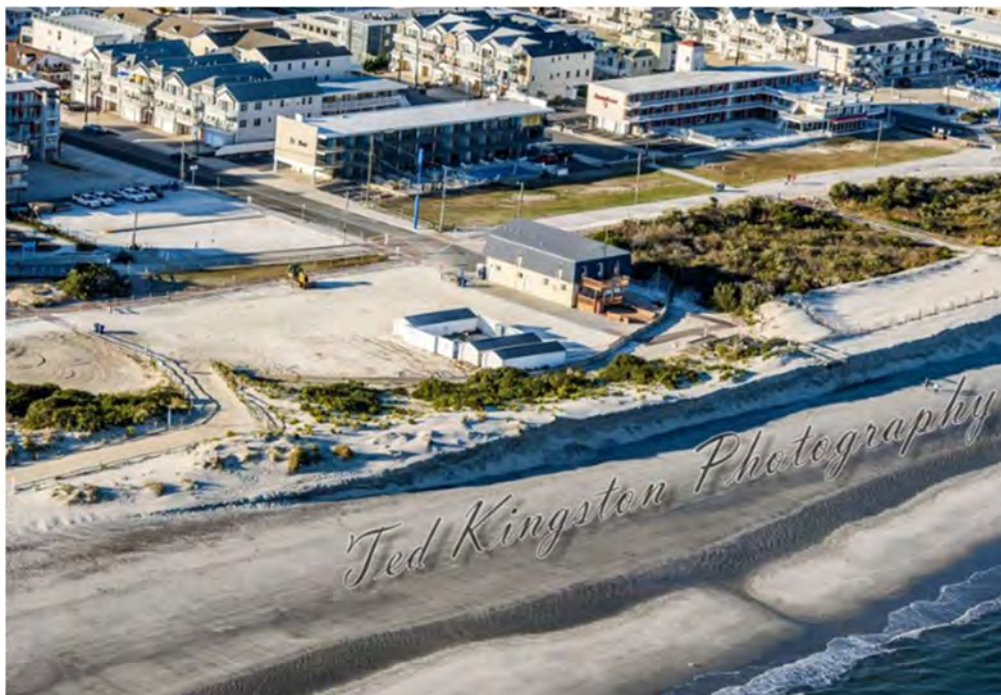
Figure 5: Drone photo depicting the erosion in the vicinity of the North Wildwood Beach Patrol Headquarters after the passage of Hurricane Ian.
