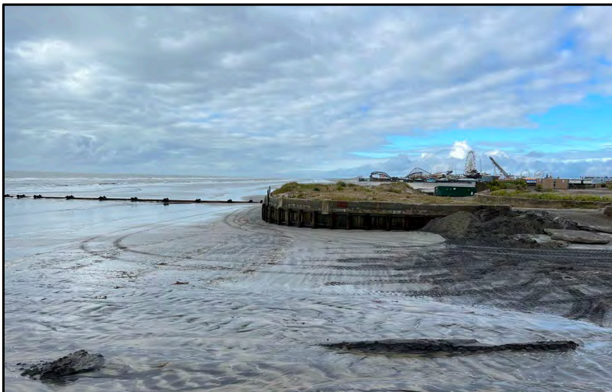
PHOTOGRAPH 4. View south of the City of Wildwood exposed stormwater outfall at the Poplar Avenue right-of-way alignment, which precludes the sand backpassing route.
