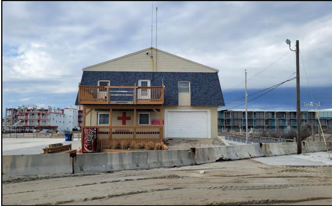
PHOTOGRAPH 5. View northwest of the deployed jersey barriers in front of the City of North Wildwood Beach Patrol headquarters authorized through an Emergency Authorization submitted on October 5, 2022
