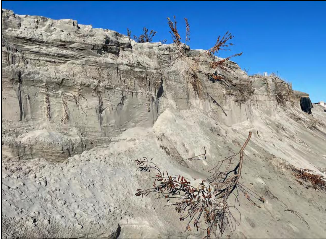
PHOTOGRAPH 3. View north of dune scarp conditions in January 2023. Note the damaged dune vegetation and negative ecological impacts of erosion.
