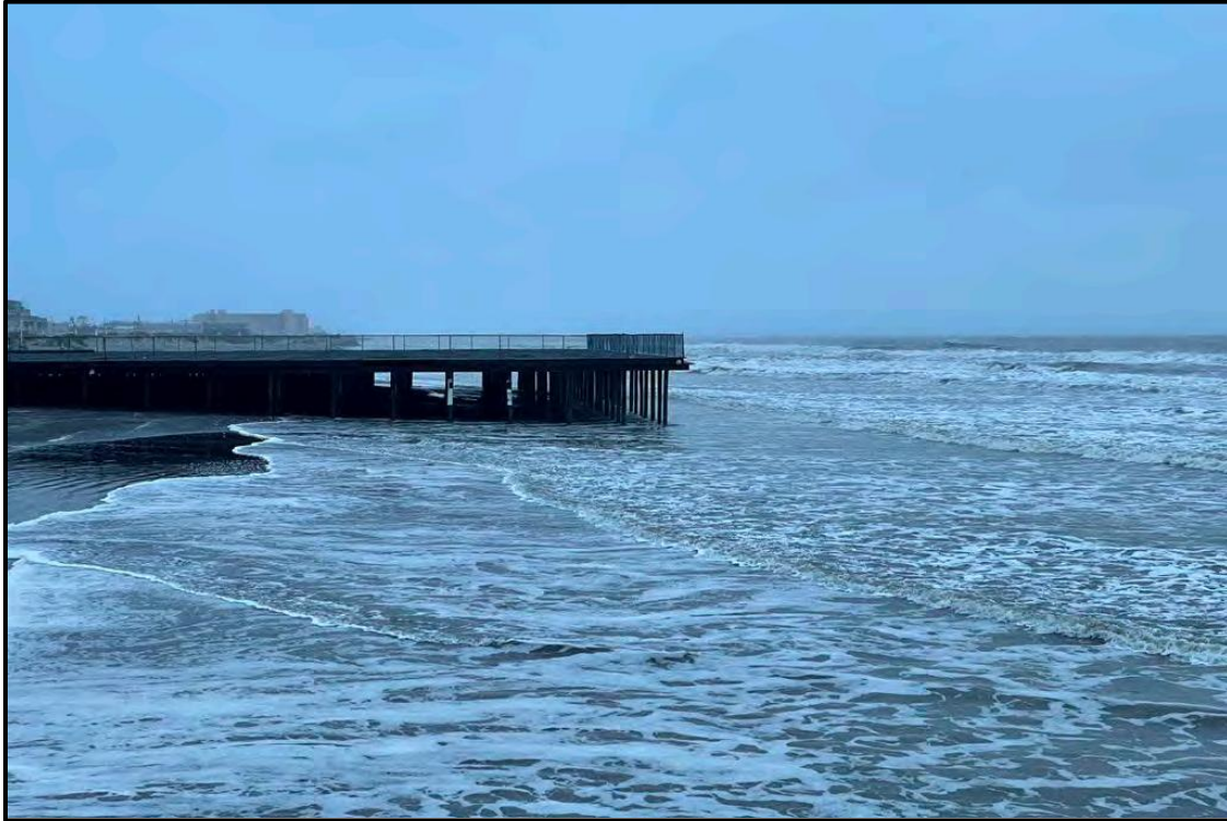
PHOTOGRAPH 7. View north of the 24 th Avenue pier terminus and absence of beach berm waterward of the pier end, which precludes the sand backpassing truck route.
