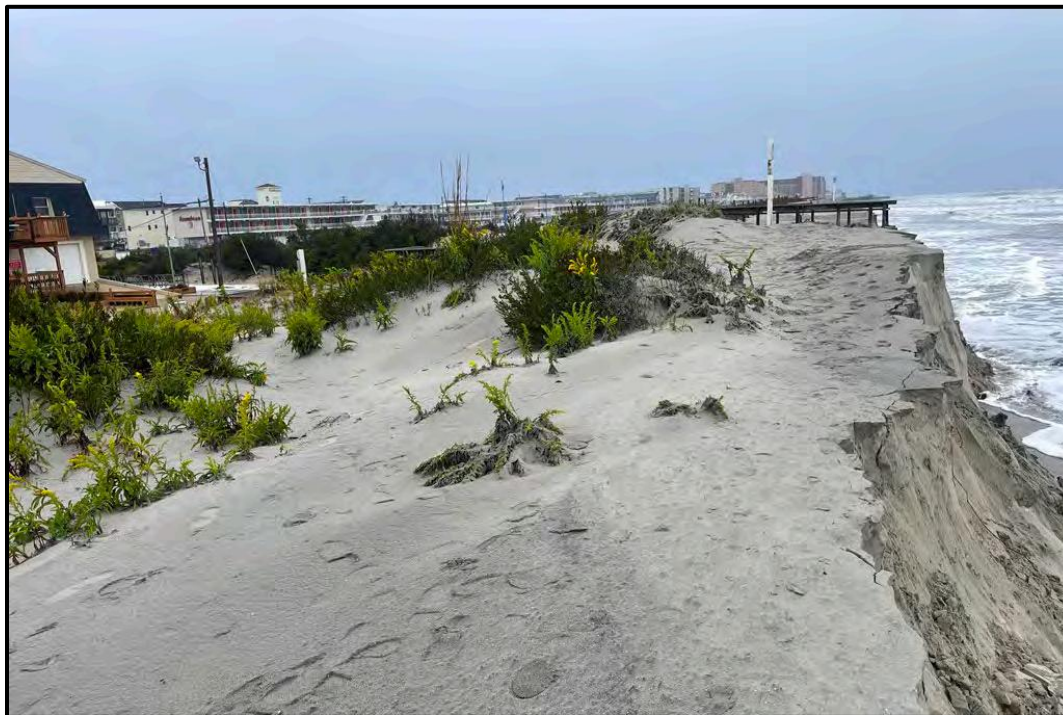
PHOTOGRAPH 1. View north of the dune scarp (right) in October 2022, during the offshore passage of hurricane Ian, eroded to a point landward of the pre-existing dune crest between 15 th and 16 th Avenues in front of the City of North Wildwood Beach Patrol headquarters (left) and upper landing of dune walkover railing (background)
