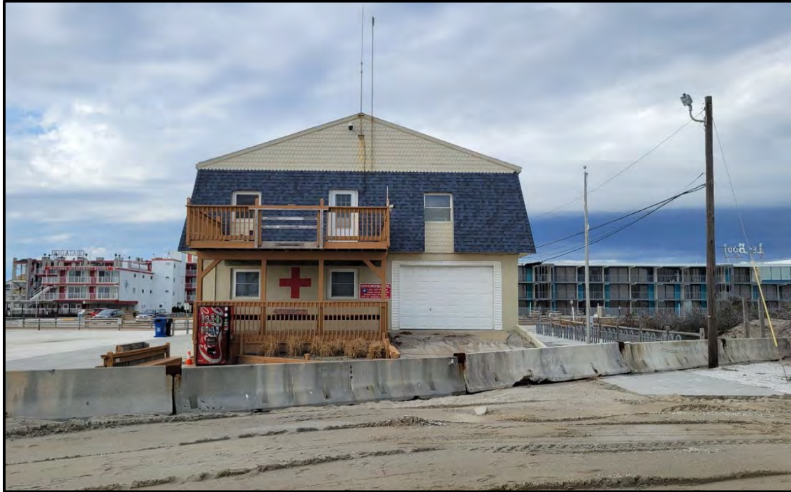
PHOTOGRAPH 5. View northwest of the deployed jersey barriers in front of the City of North Wildwood Beach Patrol headquarters authorized through an Emergency Authorization submitted on October 5, 2022
