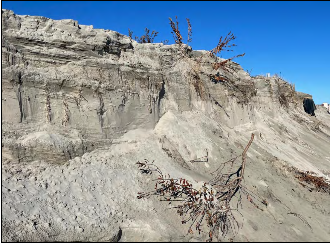
PHOTOGRAPH 3. View north of dune scarp conditions in January 2023. Note the damaged dune vegetation and negative ecological impacts of erosion.
