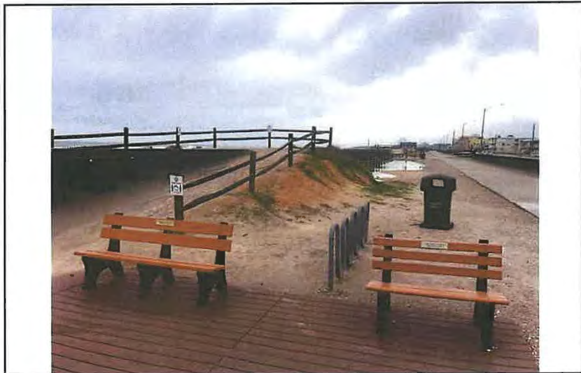
Photo #14 – View of typical beach access over steel bulkhead at 10 th Avenue looking southwest.
