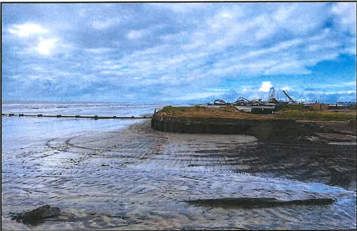
PHOTOGRAPH 4. View south of the City of Wildwood exposed stormwater outfall at the Poplar Avenue right-of-way alignment, which precludes the sand backpassing route.
