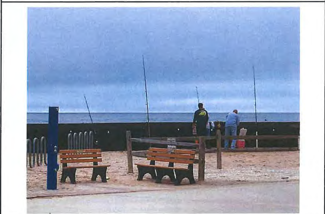
Photo #6 – View of the local community fishing at the steel bulkhead at 5th Avenue at the location of the former beach.
