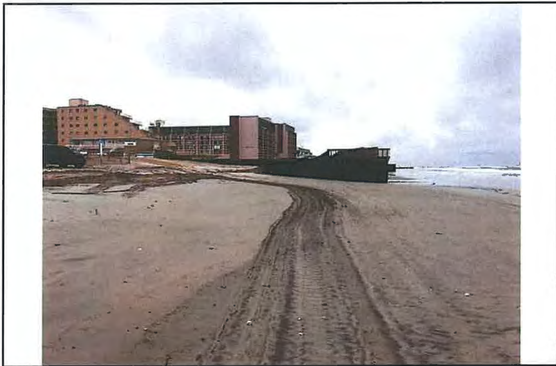
Photo #12 – View of steel bulkhead at 8 th Avenue looking northeast.
