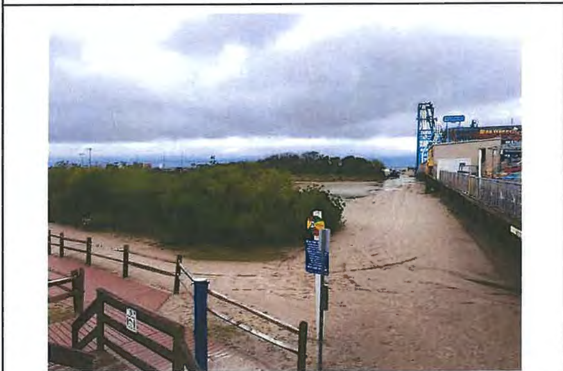
Photo #24 – View of proposed steel bulkhead location at 25 th Avenue looking southeast.
