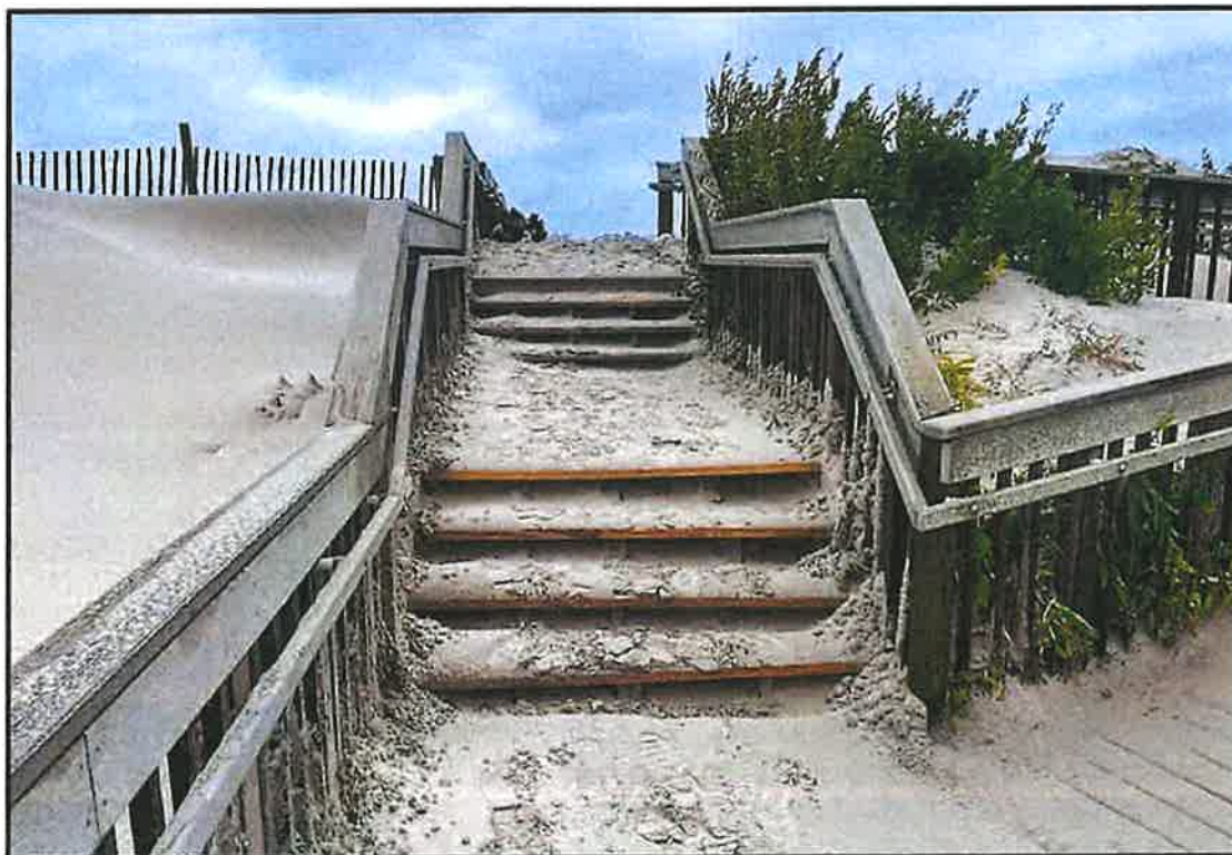
PHOTOGRAPH 6. View of the dune walkover and ADA access ramp in front of the City of North Wildwood Beach Patrol headquarters. Note: eroded dune scarp is located immediately behind the upper staircase landing.
