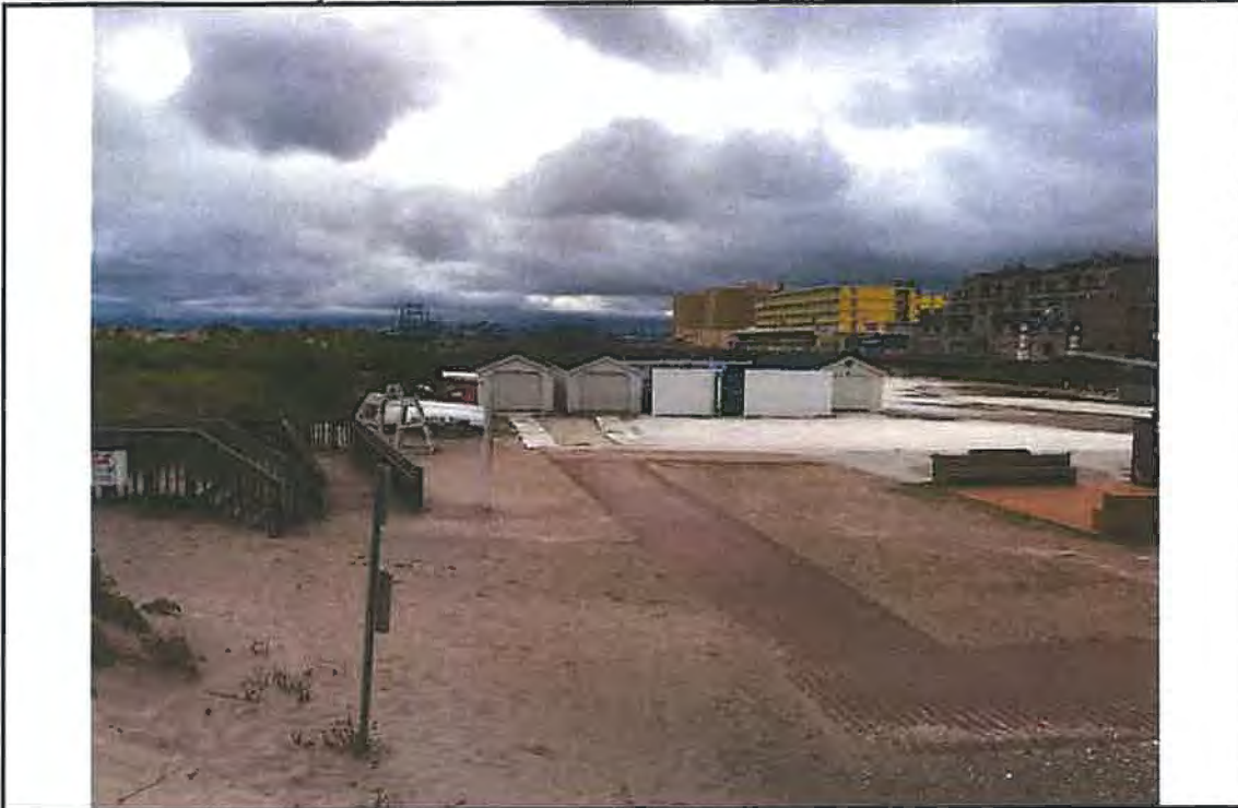
Photo #17 – View of proposed location for steel bulkhead at 15 th Avenue looking southwest near the Beach Patrol Building.
