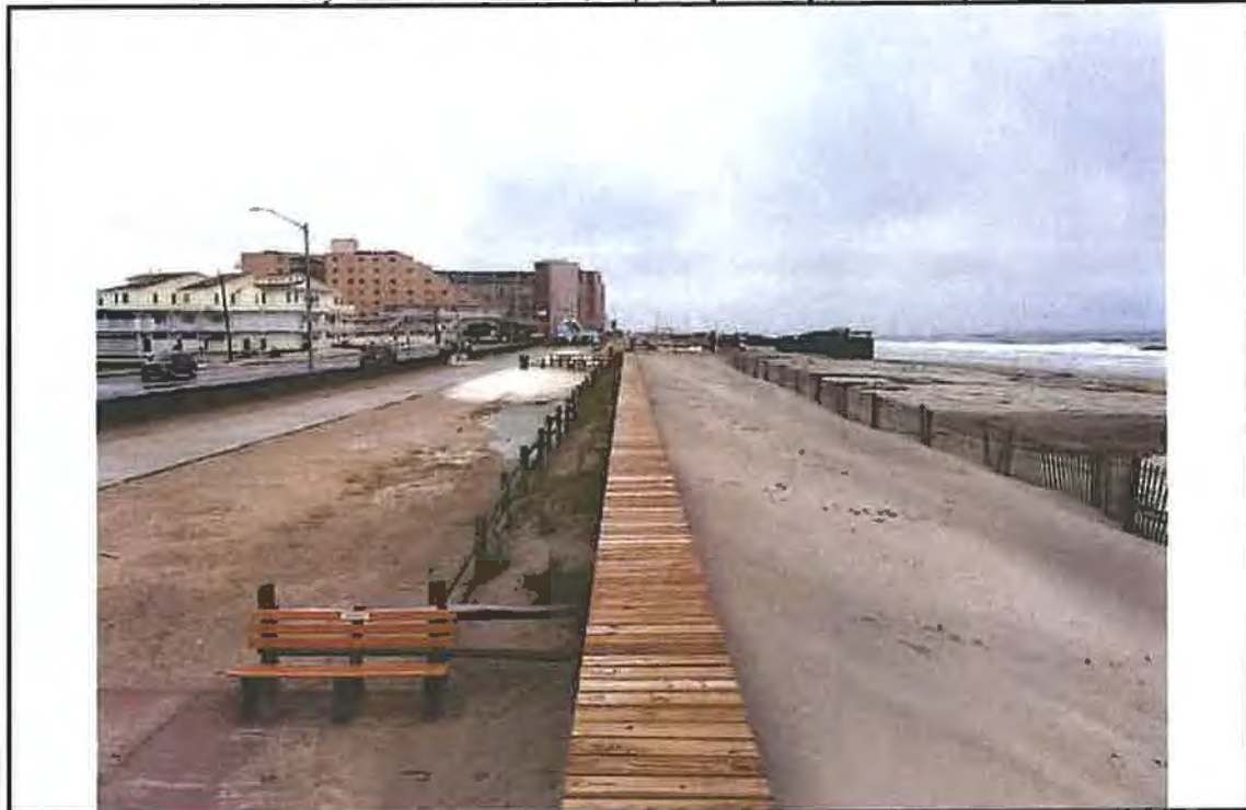
Photo #13 – View of timber cap and steel bulkhead at 9 th Avenue looking northeast showing location of former wetlands/dune.
