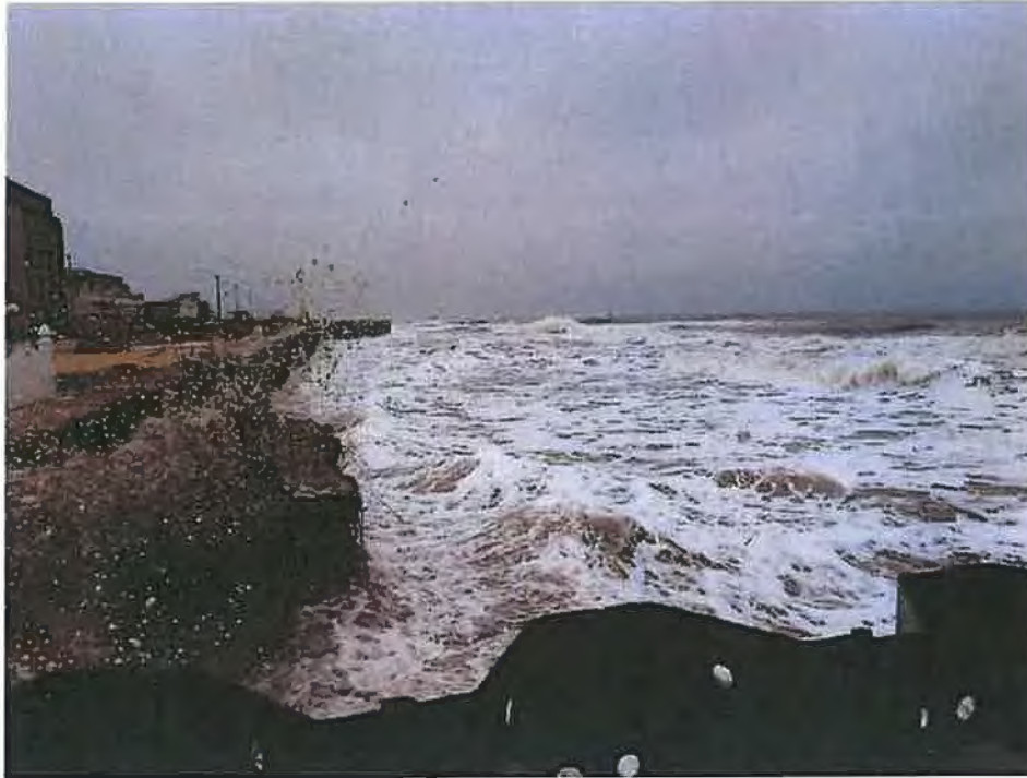
( Exhibit B , 2020 Photograph showing the emergency bulkheads from 3 rd to 13 th Avenues in action defending North Wildwood against a storm.) The dune to the lefthand side of the photo did not survive the storm, but the bulkhead behind it did.
