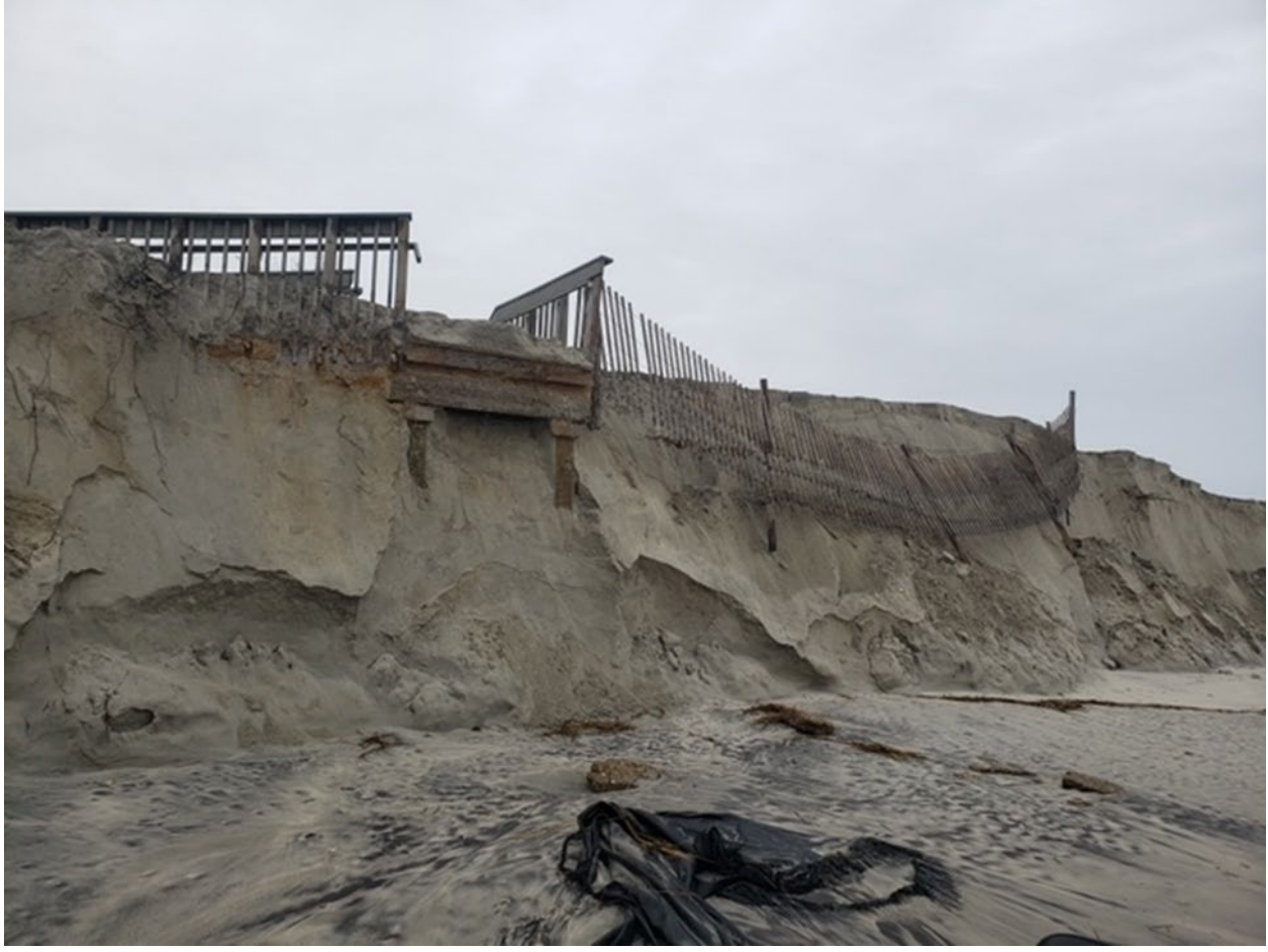
(Exhibit B, View of severe dune erosion at 15 th Avenue as of March 13, 2023.)
