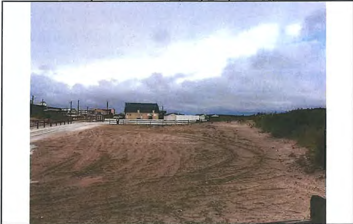
Photo #19 – View of proposed bulkhead location at 16 th Avenue looking northeast at the Beach Patrol Building.
