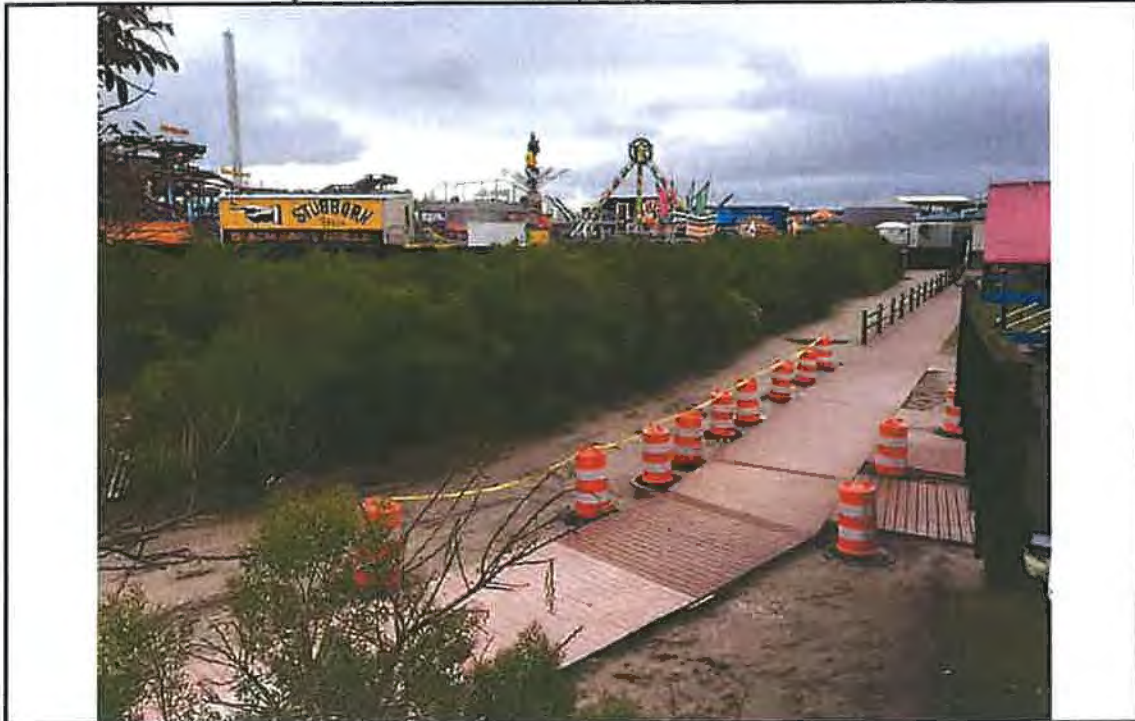
Photo #23 – View of proposed steel bulkhead location at 24 th Avenue looking southwest.
