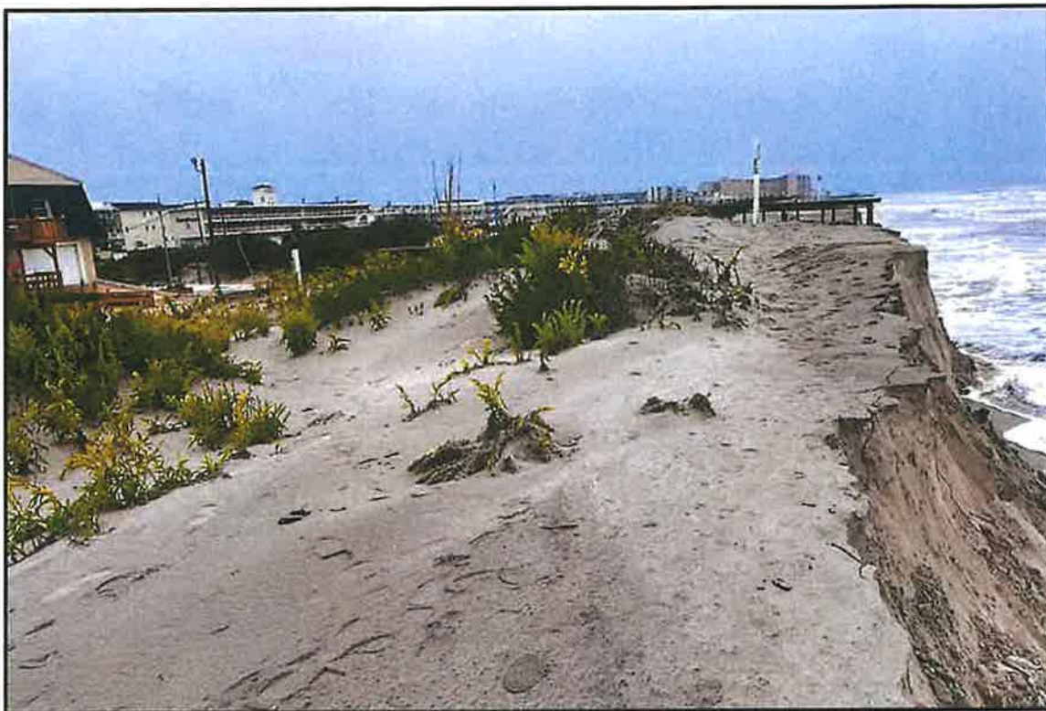
PHOTOGRAPH 1. View north of the dune scarp (right) eroded to a point landward of the pre-existing dune crest between 15 th and 16 th Avenues in front of the City of North Wildwood Beach Patrol headquarters (left) and upper landing of dune walkover railing (background)
