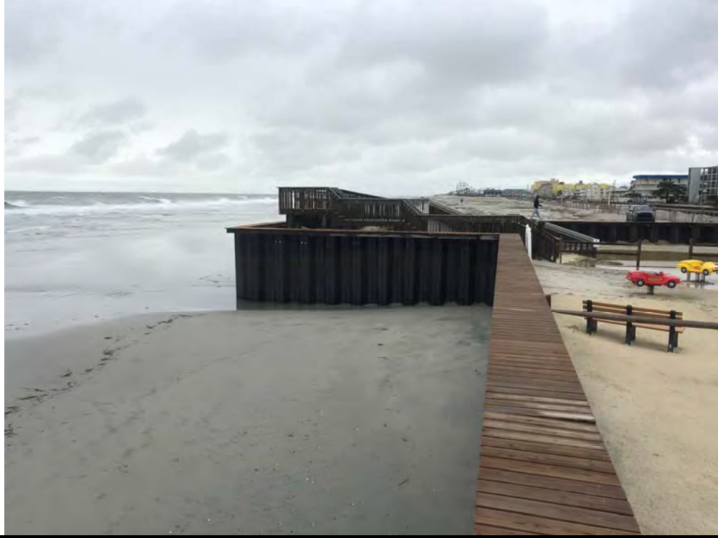
Photo #9 – View of timber cap and steel bulkhead looking southwest toward 7 th Avenue.
