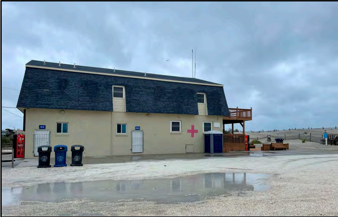
PHOTOGRAPH 5. View of the City of North Wildwood Beach Patrol headquarters which serves as a critical oceanfront safety facility with public access amenities. Note: eroded dune scarp is located at the right edge behind the dune fencing.
