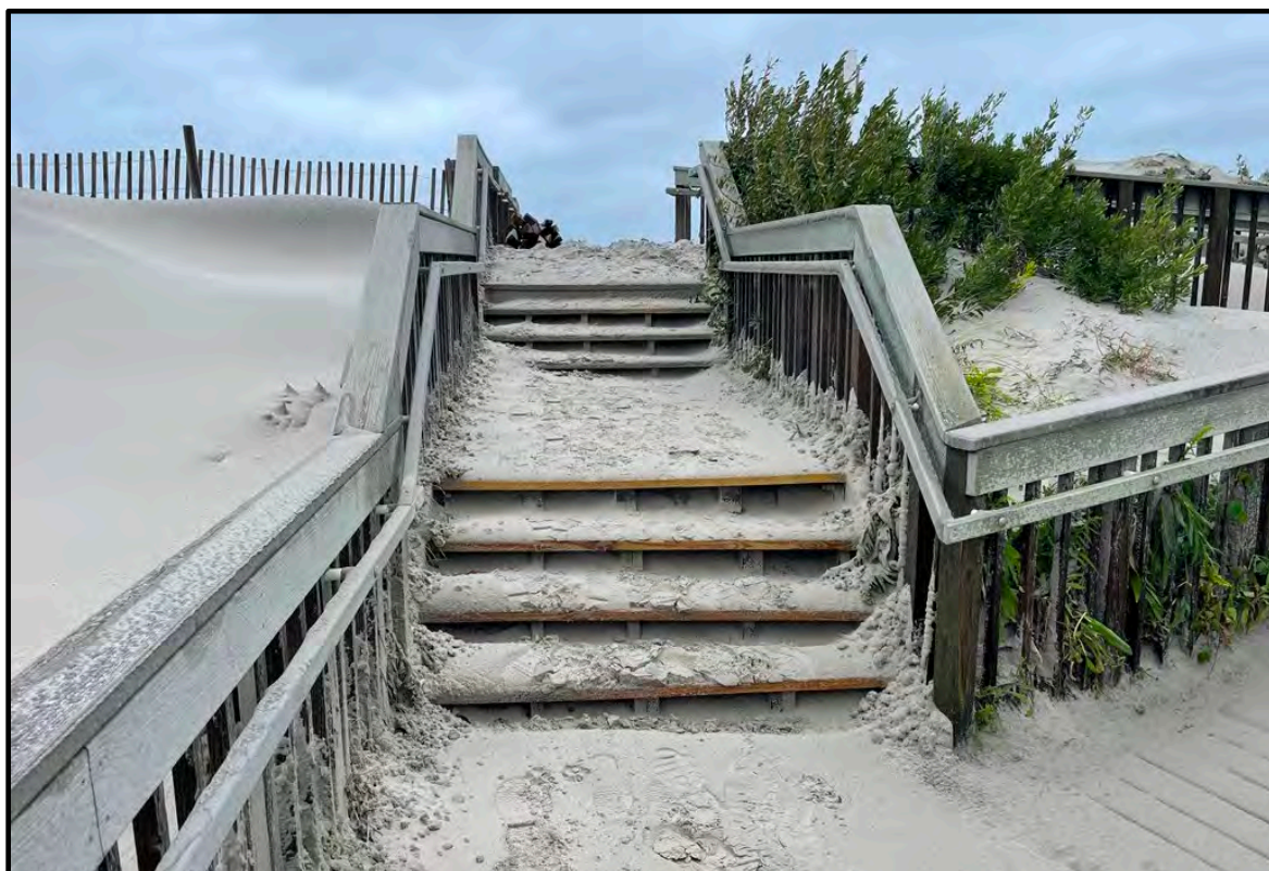
PHOTOGRAPH 6. View of the dune walkover and ADA access ramp in front of the City of North Wildwood Beach Patrol headquarters. Note: eroded dune scarp is located immediately behind the upper staircase landing.
