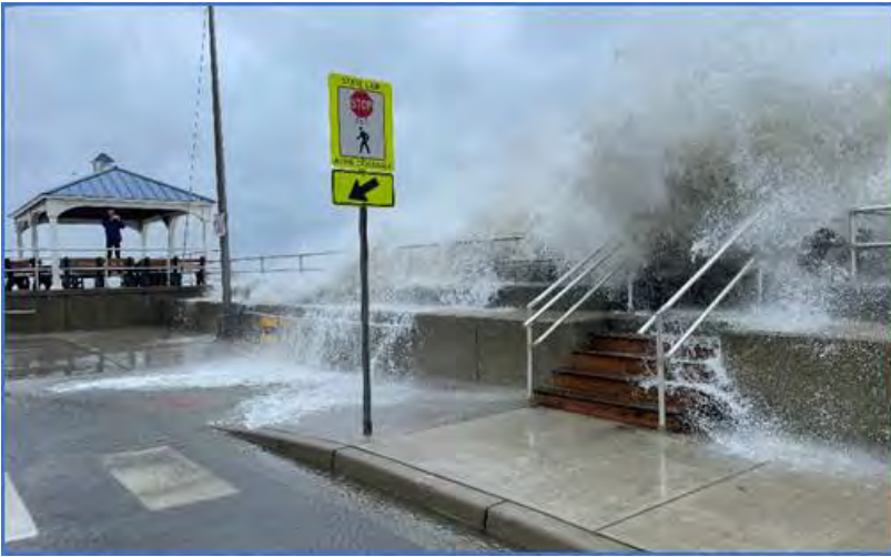
View at 3 rd Avenue/JFK Avenue seawall/stormwater outfall vent this afternoon
