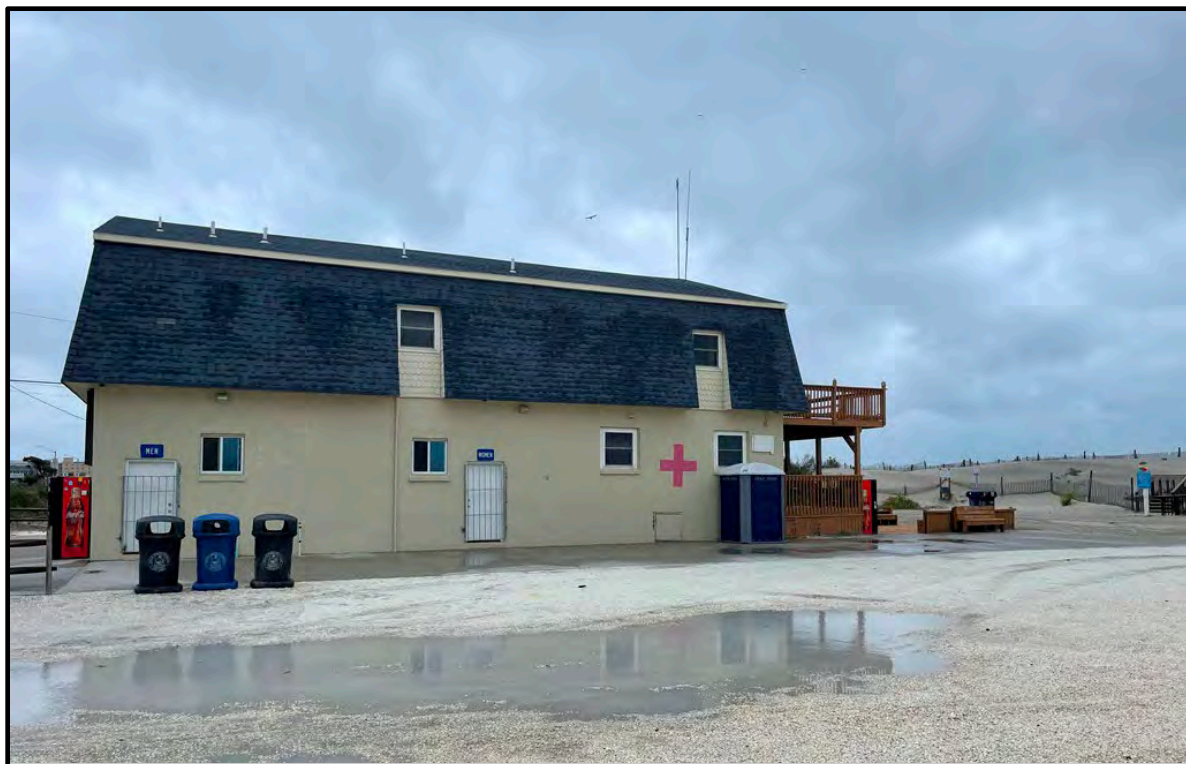
PHOTOGRAPH 5. View of the City of North Wildwood Beach Patrol headquarters which serves as a critical oceanfront safety facility with public access amenities. Note: eroded dune scarp is located at the right edge behind the dune fencing.
