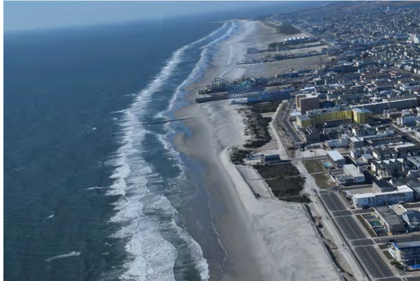
Figure 3: Aerial photograph looking south depicting the beach in the vicinity of the North Wildwood Beach Patrol Headquarters after the passage of Hurricane Ian.
