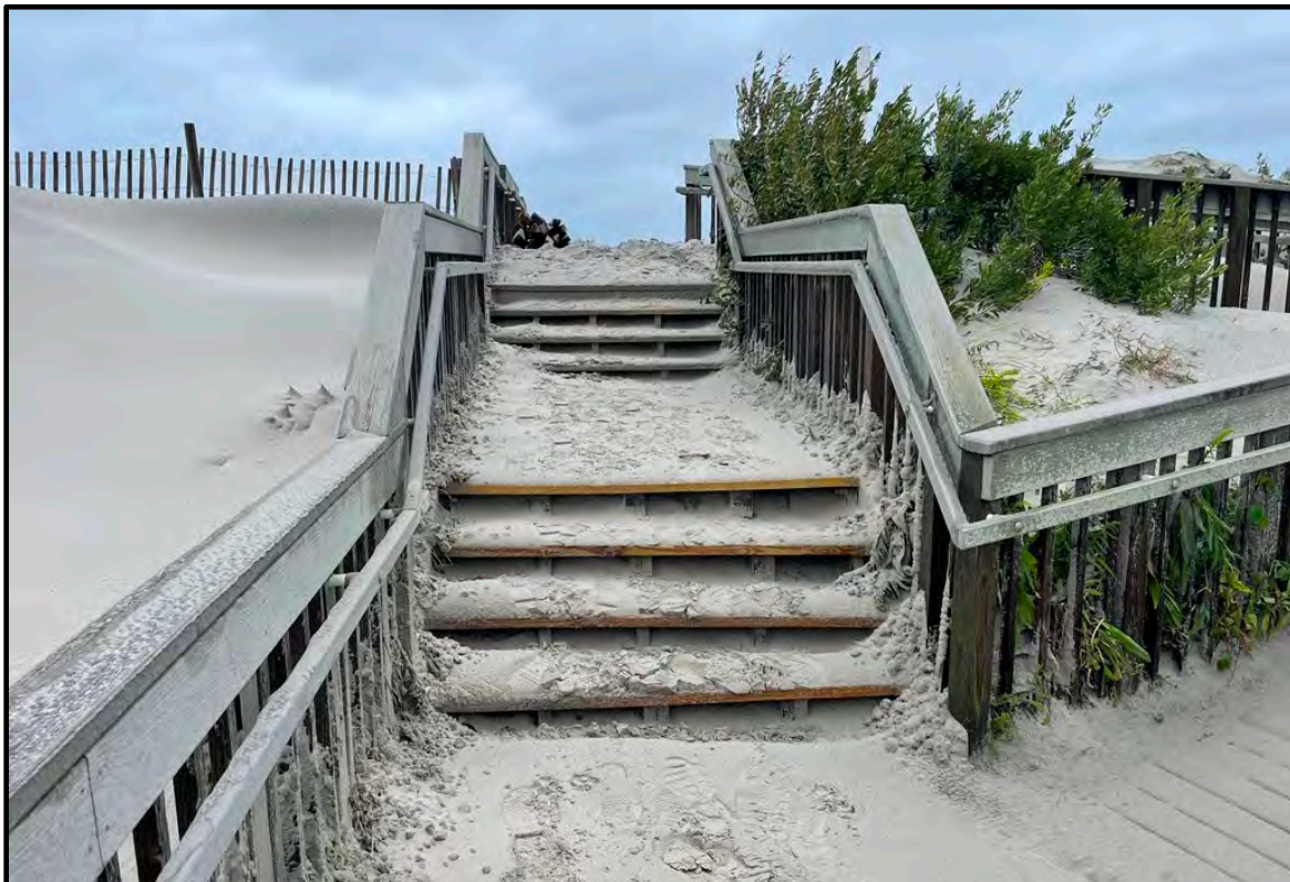
PHOTOGRAPH 6. View of the dune walkover and ADA access ramp in front of the City of North Wildwood Beach Patrol headquarters. Note: eroded dune scarp is located immediately behind the upper staircase landing.
