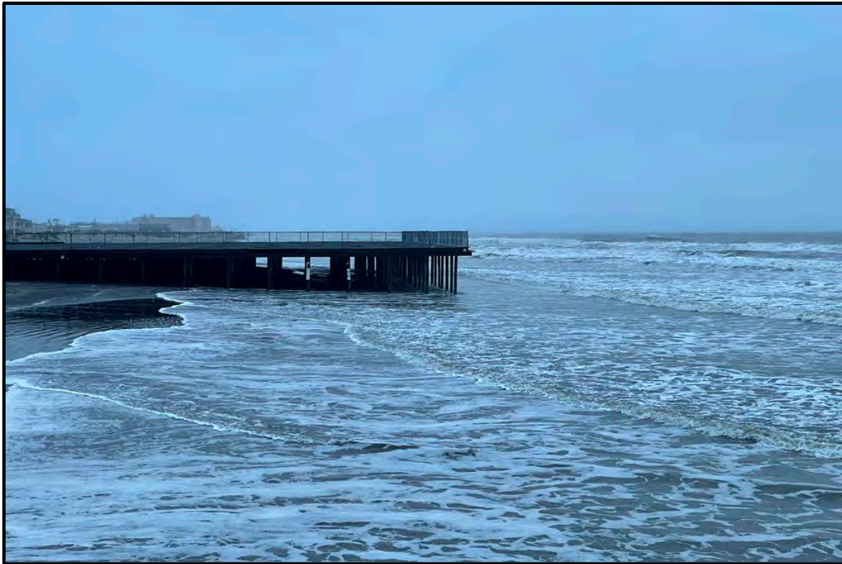
PHOTOGRAPH 3. View north of the 24 th Avenue pier terminus and absence of beach berm waterward of the pier end, which precludes the sand backpassing truck route.
