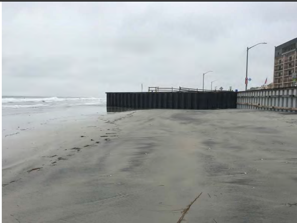
Photo #4 – View of waterward side of vinyl bulkhead and steel bulkhead, and former dune area at 4 th Avenue looking southwest.
