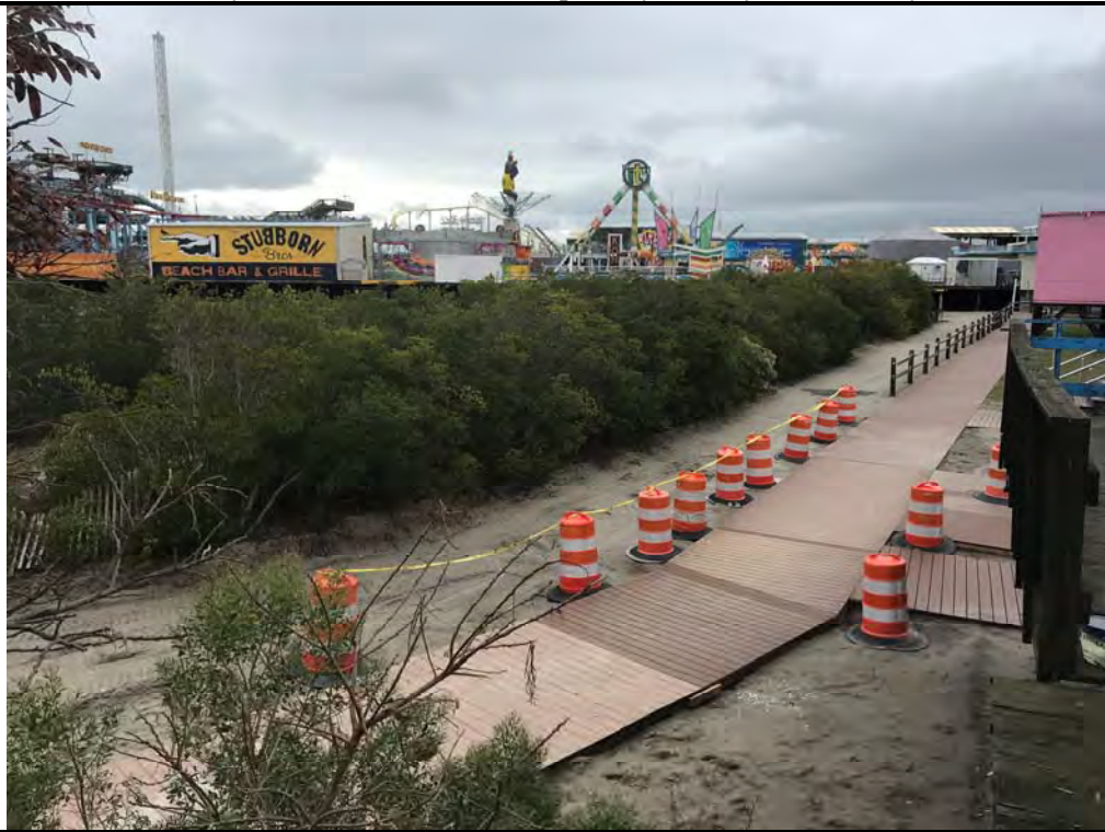
Photo #23 – View of proposed steel bulkhead location at 24 th Avenue looking southwest.
