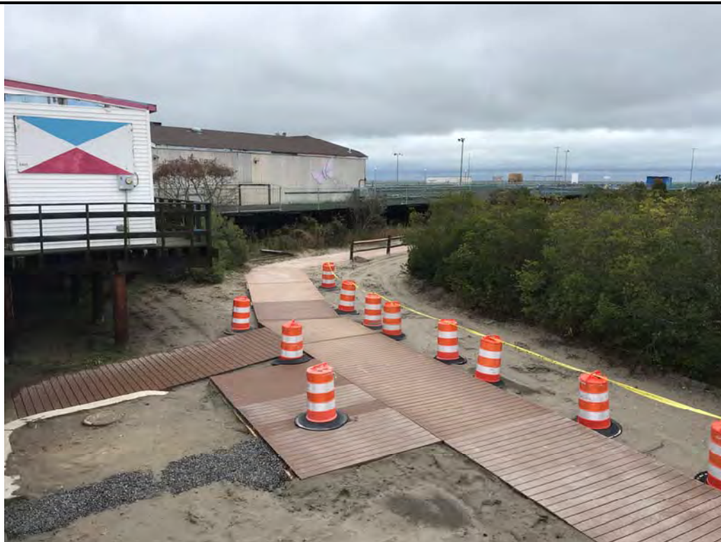
Photo #22 – View of proposed bulkhead location at 24 th Avenue looking southeast.
