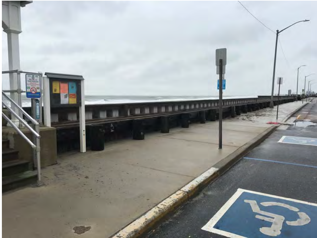
Photo #1 – View of landward side of vinyl bulkhead at 3 rd Avenue looking southwest.
