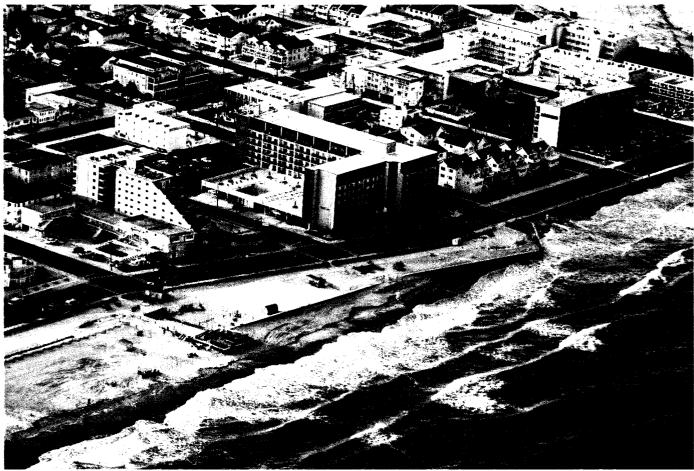
Figure 2. This June 2023, photograph shows the waves impacting the revetment along JFK from 6<sup>th</sup> Avenue north to the inlet. A narrow strip of sand at high tide from 6<sup>th</sup> Avenue south widens past the handicap ramp to support a small dune. (Aerial Photo by Ted Kingston for CRC)
