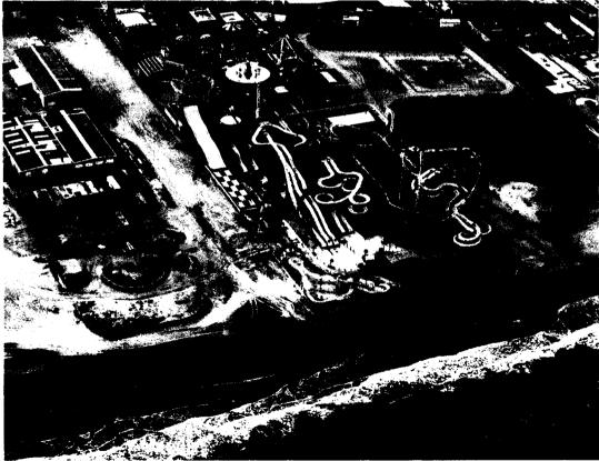
Figure 24. The aerial photo above was taken on May 22, 2023, view is looking onshore at the ends of the two piers adjacent to the profile. An intertidal (wet) beach exists at the steel bulkhead protecting the amusement pier and water park from the ocean with a massive dry beach extending well landward to the boardwalk providing protection for boardwalk and community. This site is adjacent to the municipal border with Wildwood.
